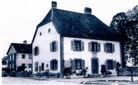
Pavilion next to the Logis de la Licorne Gagnebin House
