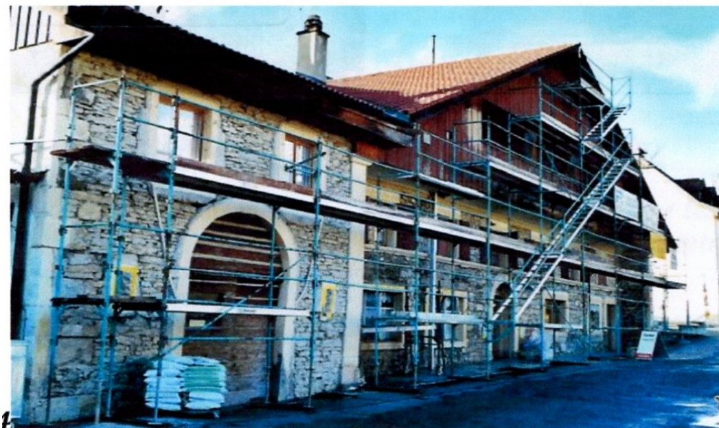
April 2001 Renovation of the façade
