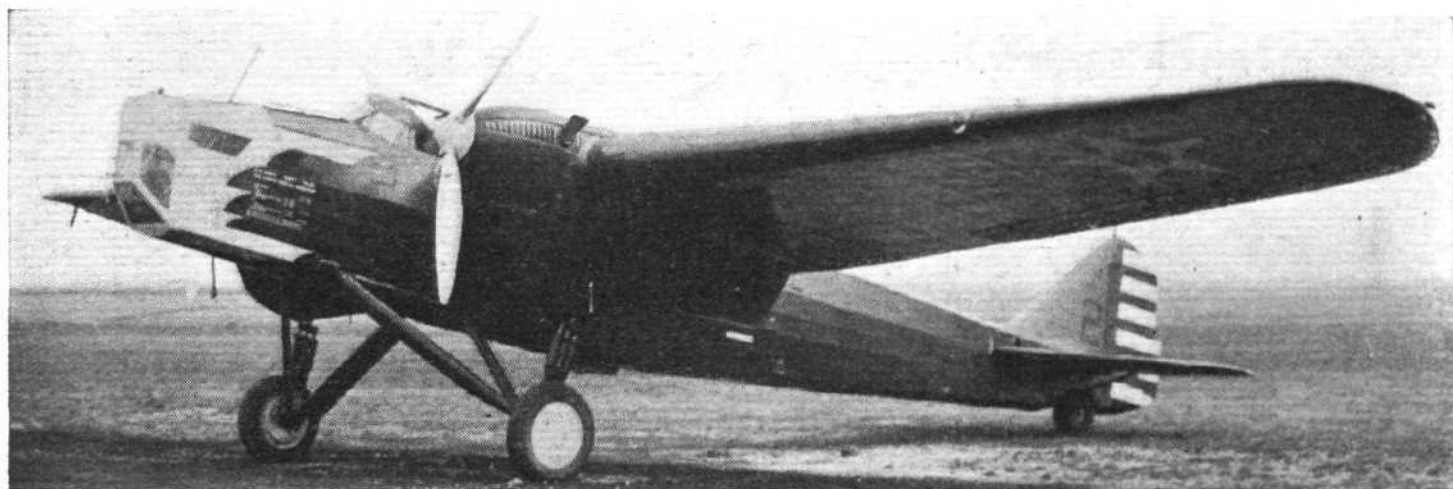
FOR ARMY OBSERVATION: The Fokker o-27 is designed for long-range reconnaissance. It is fitted with two Curtiss "Conqueror" engines of 650 h.p. each.
